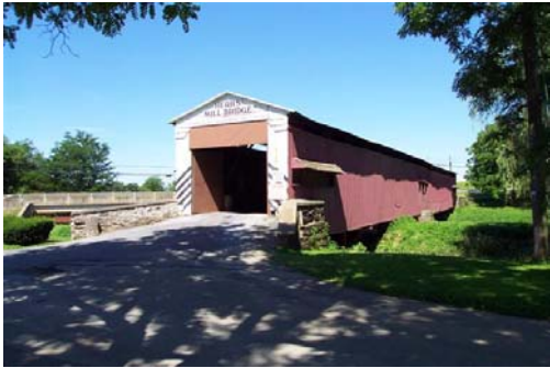
Mill Covered Bridge, Pequea Creek, Lancaster
