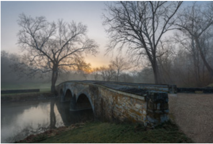
Burnside Bridge at Dawn, © Alan Sislen
